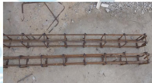
Figure 1: Steel Reinforcement for the beam
