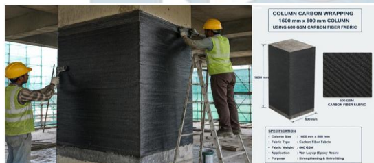
Figure 5: Column Strengthening by Carbon Fiber Wrapping
