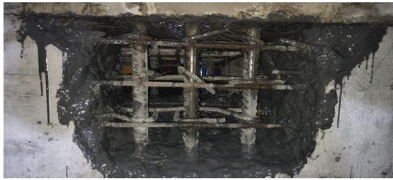
Figure 2: Column top Dismantled partwise
