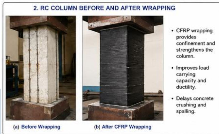
Figure 4: RC Column before and after wrapping
