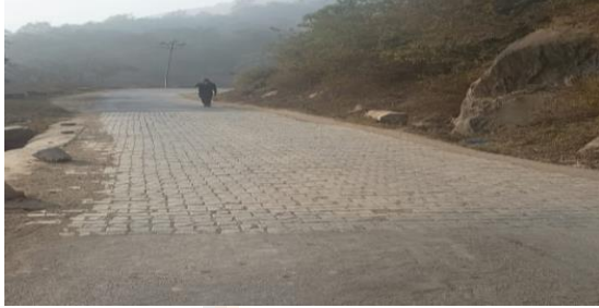
Figure 7: Paver Block Road
