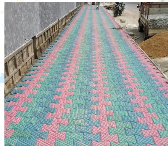
Figure 3: Paver Blocks for footpath Kerb
