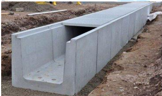
Figure 5: Road Side Drainage
